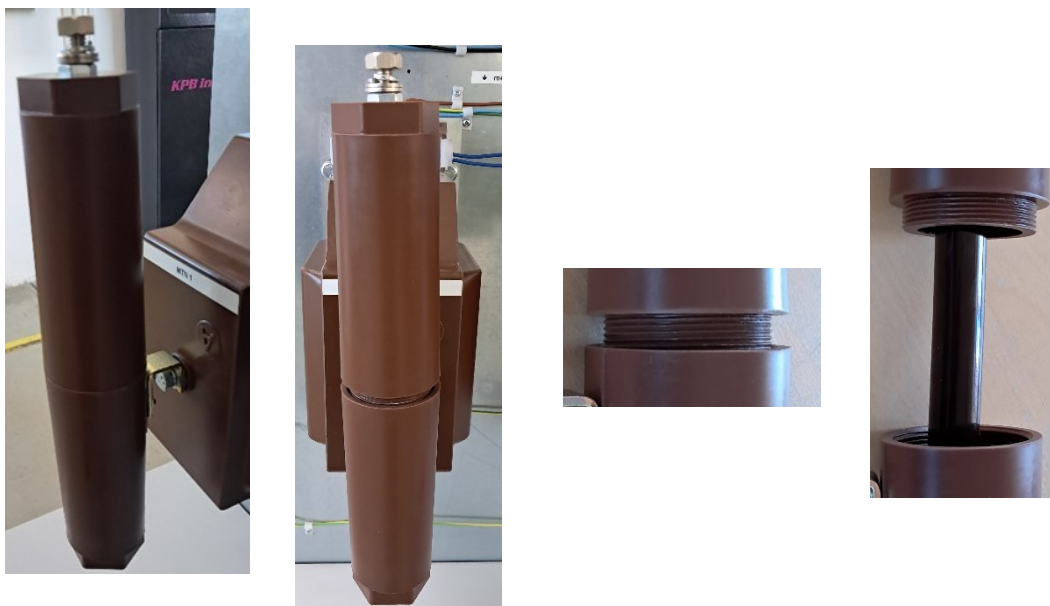
Figure 8: Procedure for removing the fuse insert (cartridge) from the fuse case
