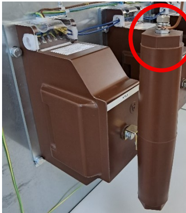
Figure 2: Marking the location of the HV part disconnection
